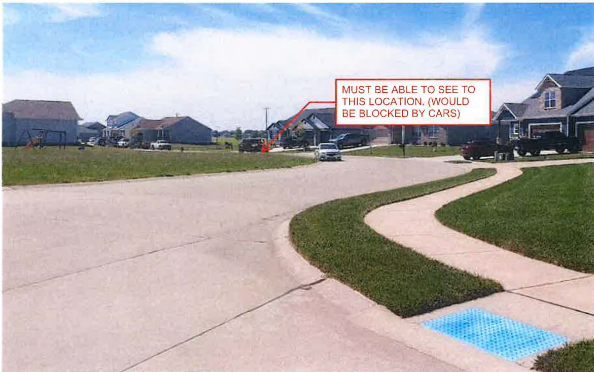
Photo 2: Sight-triangle looking north along Eisenhower from eastern approach of intersection.
